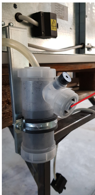
5. picture: Installation of condensate drain siphon
